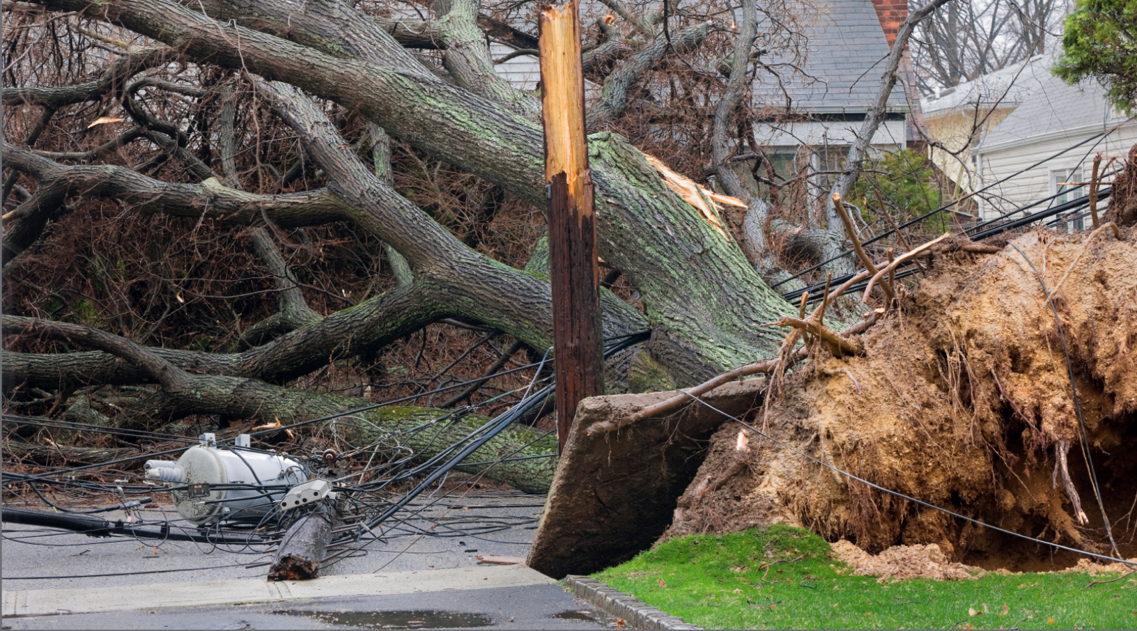
Damage caused by a hurricane
