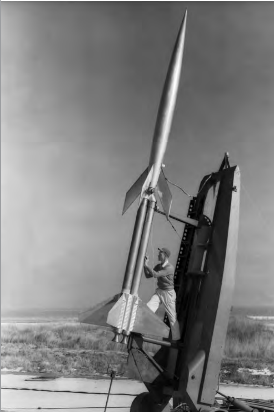
Technician Durwood Dereng measures elevation of double Deacon booster prior to launch of RM-10 research model at Wallops, February 6, 1951.
